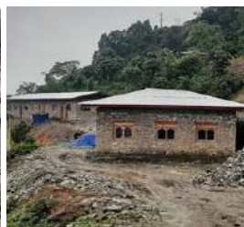
Construction of BHU II at Kamji
