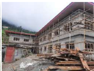
Staff quarter construction at Gedu
