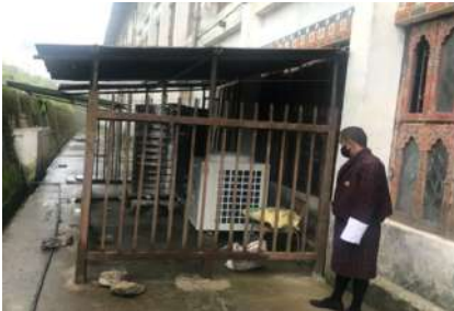
Heating System Installation at Chhukha CS
