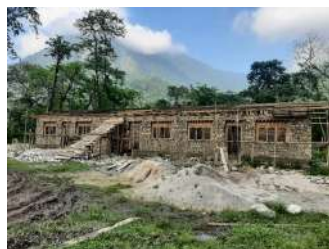
BHU staff quarter at Piping
